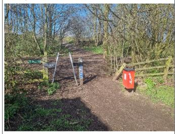
Current A frame width (Top Width - 36cm Bottom Width -100cm) is not compliant with Equality Act 2010 and restricts some legitimate users in wheelchairs, mobility scooters and adapted cycles.
