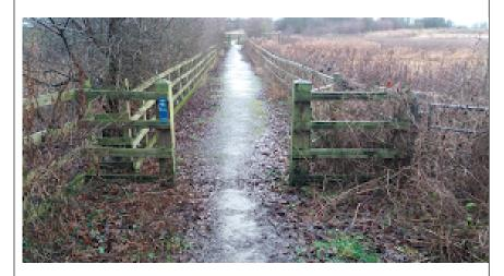
Access control widened to leave a gap of 1.6 meters ensuring compliant gap for Equestrian users, cycles and pedestrians. Path width 2 meters following access
