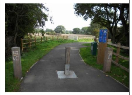
Access control widened to leave two gaps of 1.6 meters ensuring compliant gap for Equestrian users, cycles and pedestrians. Path width 4 meters following access
